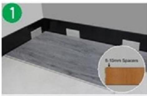
Provide a 6mm – 10mm expansion gap between the floor and your walls or fixed objects. This is the allowance for minimal expansion rate of +/- 0.1% average
