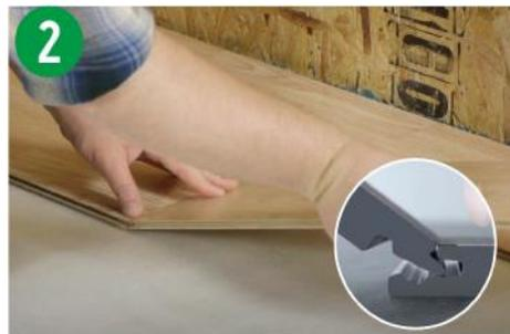
Match the long edge first, keep +/- 20° angle when inserting.
