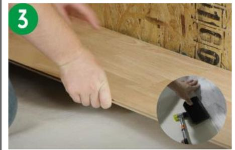
Use a rubber mallet to gently lock the short edge, use a tapping block to fasten the locking system.
