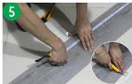
Cut both sides of the plank using utility knife and a square ruler to make sure the cutting edge is straight.
