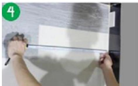
Measure the length of end plank for the row, the length must have a minimum of 30cm. You may need to shorten the first piece for the row.
